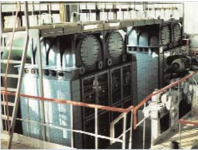
Figure 22. UV drinking water plant 405.000 m 3 per day, Tollyaytti (Russia).
